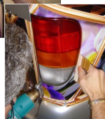
It is very important to 'heat-set' (re-cast) the film in channels and swages. It's also advisable to do this with edges and curves, to avoid curling.
