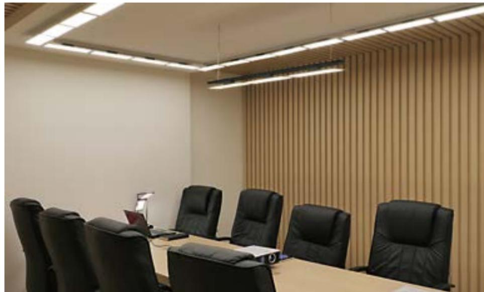
Track lights with OLEDs can be connected to commercially available tracks.
