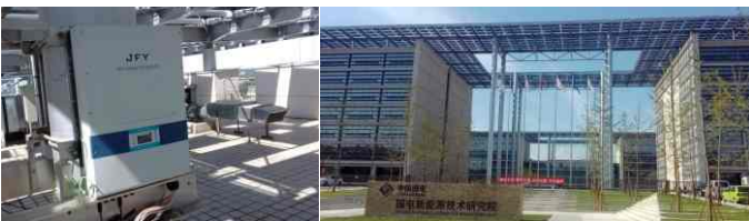
Guodian 2.58MW Photovoltaic Project in Beijing
