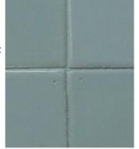
This will provide an irregular joint. Sometimes tiles have to be turned 90 degrees because no tile is the <sup>2</sup> same size. For a sharp joint, use a slightly wet sponge to clean the joints, the sharp edges of the tiles will then be noticeable.
