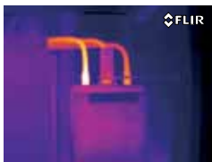
Poor connection and internal damage
