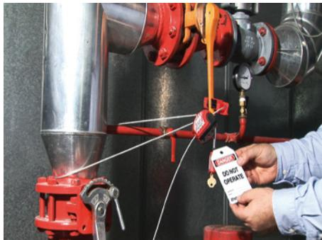
Innovation from Master Lock, the cable S806 is infinitely adjustable and fits all lockout application types.
