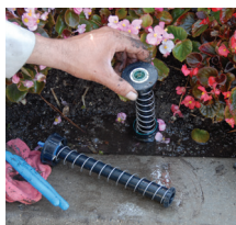
Remove the "guts" of 1806 spray head
