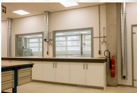
Wet Lay-Up room - Fume extraction ducts
